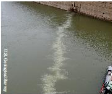
The air-bubble curtain, visible when the BAFF is turned on.
