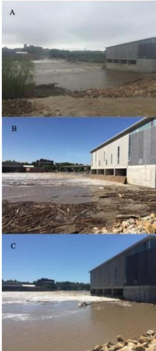
Figure 3: Water levels at Bowersock Dam during discharge events in the summer of 2019. Pictures show discharges of (A) ~15,000 cubic feet per second (cfs), (B) ~ 70,000 cfs and (C) ~ 98,000 cfs.
