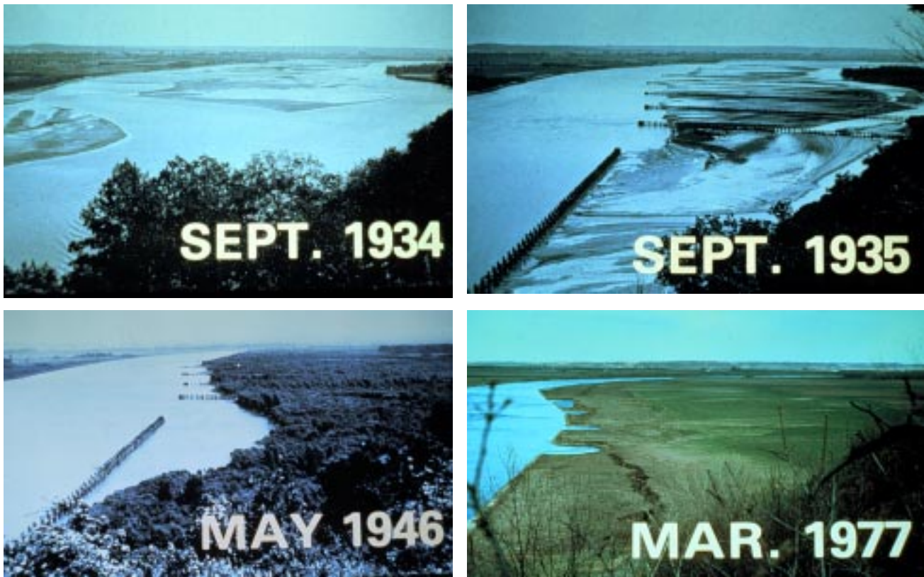
Figure 2. Development of the lower Missouri River for commercial navigation and flood control. Photos courtesy of the Missouri Department of Conservation.
