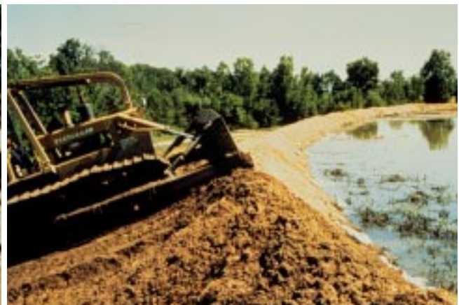
Figure 5. The raising of this federal agricultural levee during the 1993 “flood fight” threatened neighboring lands by further constricting the floodplain and forcing flood waters to higher elevations. Photos courtesy of the U.S. Fish and Wildlife Service.
