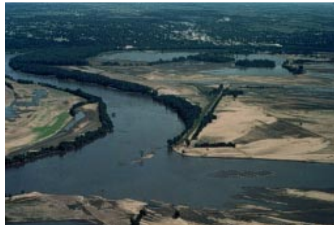
Figure 10. Missouri River levee break.
