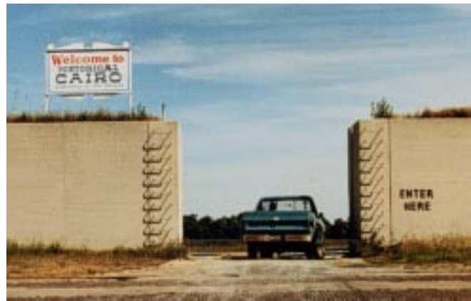
Figure 8. The floodwall at Cairo, IL isolates the city from the Mississippi River - the very reason for its establishment in the first place.
